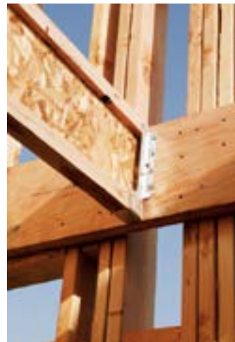
Face mount hangers can accommodate the variable depths of Tapered Red-I™ joists.
