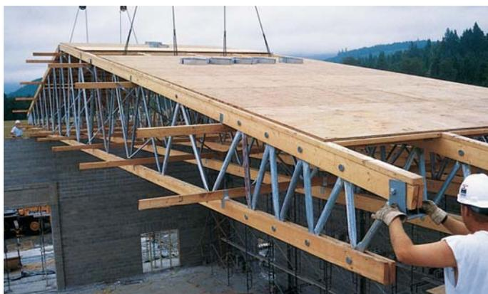
These heavy-duty, long-span pitched trusses are installed modularly.
