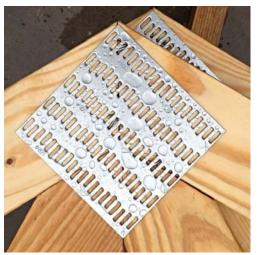
Example of a metal plate-connected truss. Photo credit: Truss Plate Institute
