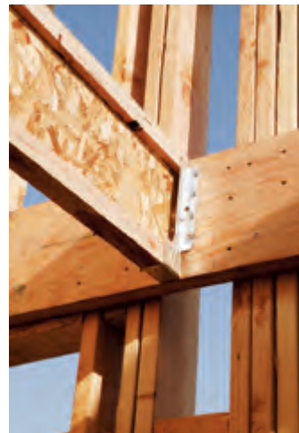
Face mount hangers can accommodate the variable depths of Tapered Red-I™ joists.
