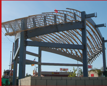
Open-web trusses allow for greater architectural flexibility, such as the curved roof of this quick-service restaurant in California.
