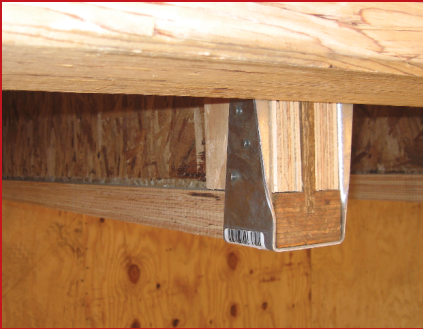
Factory-attached web stiffeners.
