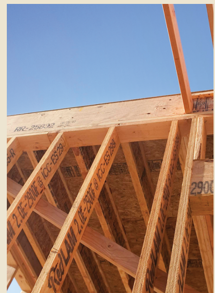
RedLam™ LVL provides support in applications throughout a structure.
