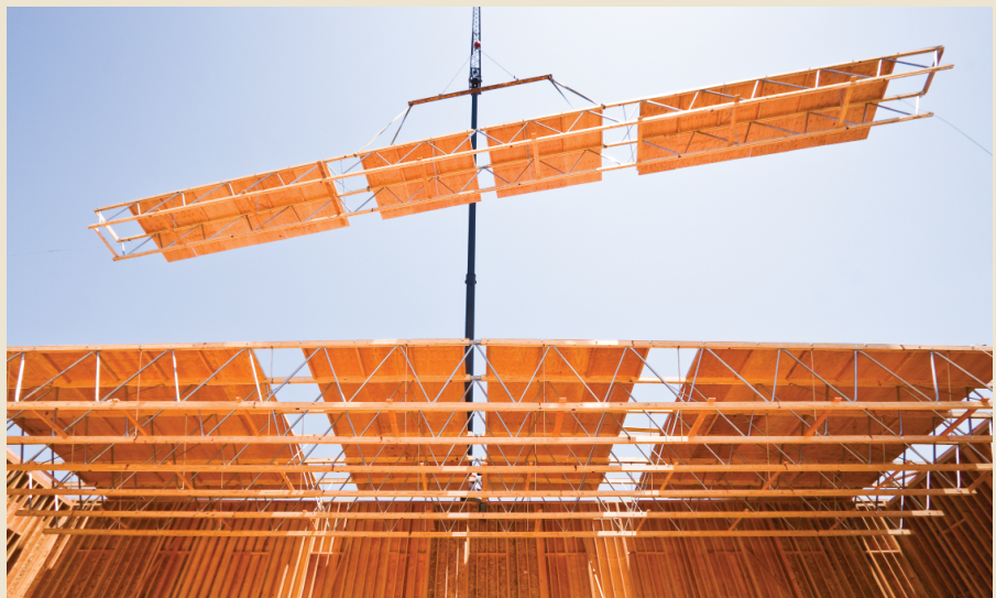
Long-span trusses are an excellent solution where uninterrupted space is necessary, such as in this church's multi-purpose building.
