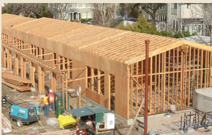
Clean, straight roof lines are the standard with Red-I™ joists, as demonstrated in this school building in California.
