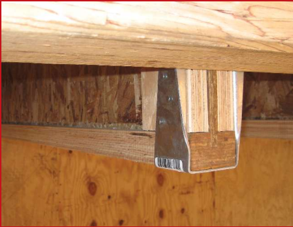
Factory-attached web stiffeners.
