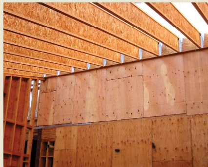
Red-I™ joists offer the workability of wood for fast, easy installation using traditional framing tools.
