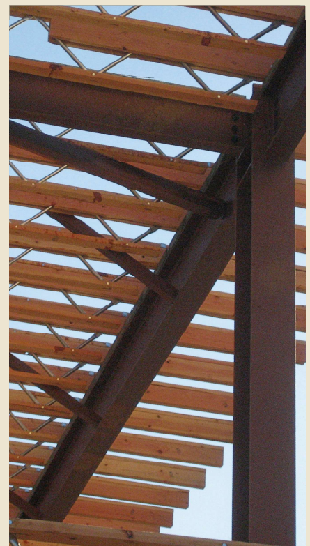
Open-web trusses can be delivered with outriggers pre-assembled, such as in this LEED®-certified professional building.
