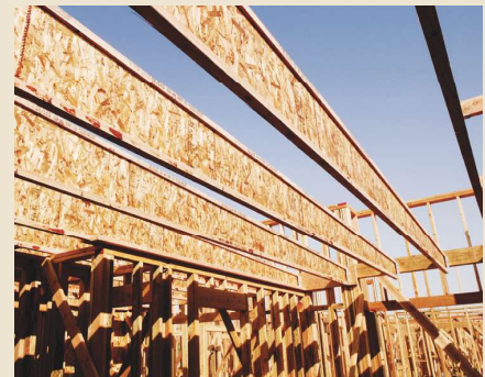
Red-I™ joists provide for longer spans, opening up floor space for more efficient use.
